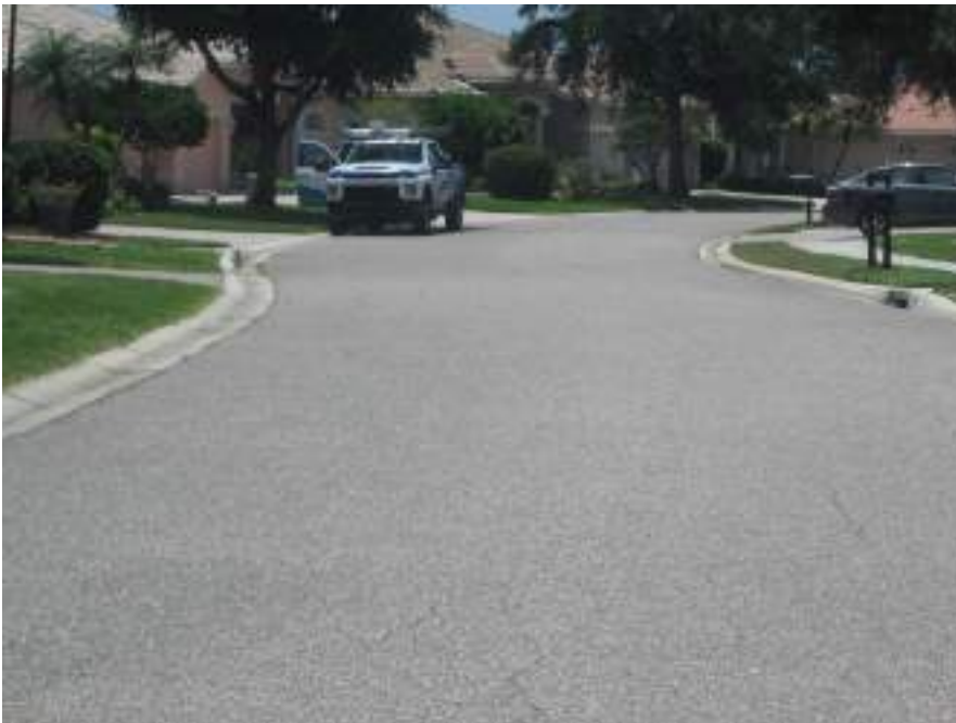
Southwest side of Camden Harbour drive viewing west
