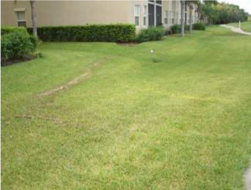
High Water Mark on sod behind condo's
